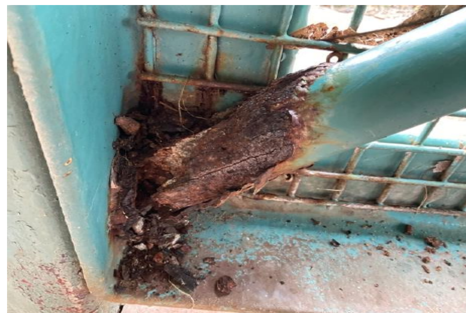
TYPICAL RUSTED COLUMNS
